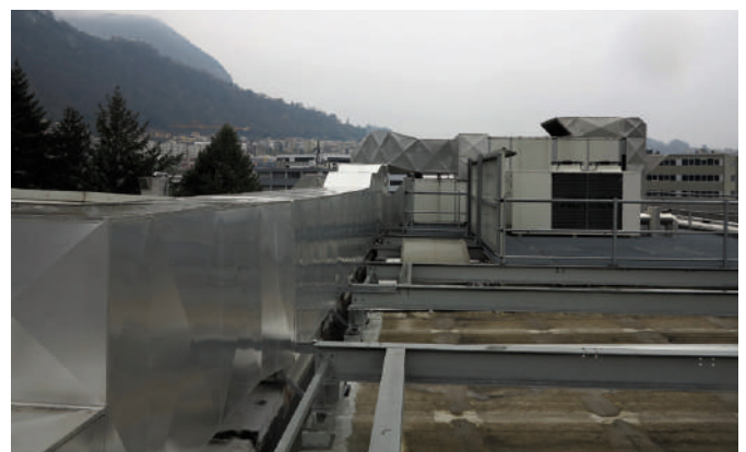
Roof-mounted ventilation system. Photo: Márton Varga, Topmotors
